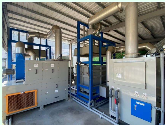
▲ Catcher's Sludge Drying System
